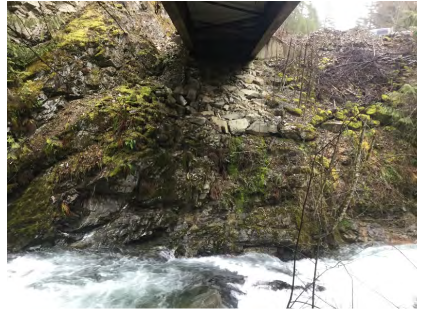
Left Bank Abutment when facing downstream
